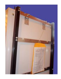
Figure 5.10.: Clamping claws and mounting brackets
