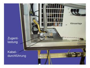
Figure 5.17.: Cable passage and strain relief
